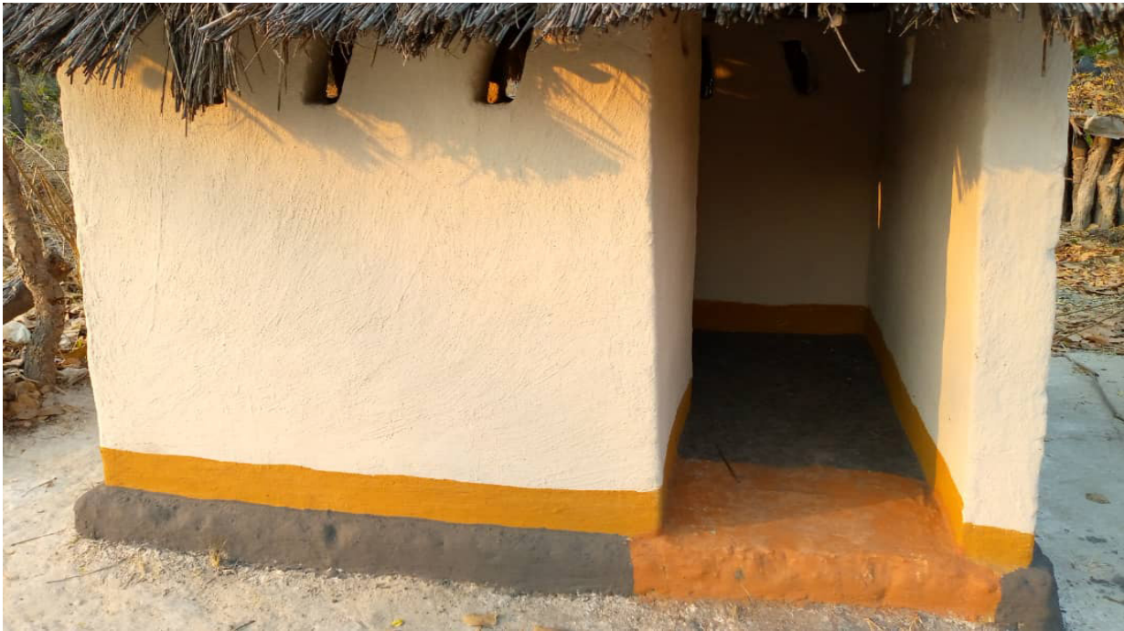
Construction of latrines increases hygiene and sanitation in communities
