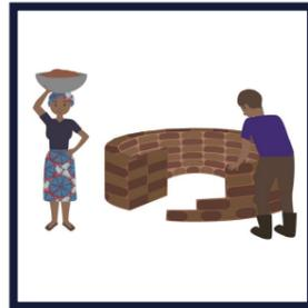
**Construct** the 1 meter wall structure from foundation by mixing anthill soil with water.
